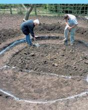
• If using a flexible liner, place a layer of builder's sand over the sides and base or use a pool underlay mat or domestic rubberbacked carpet. These help prevent the liner from being punctured. Use a good quality liner.
